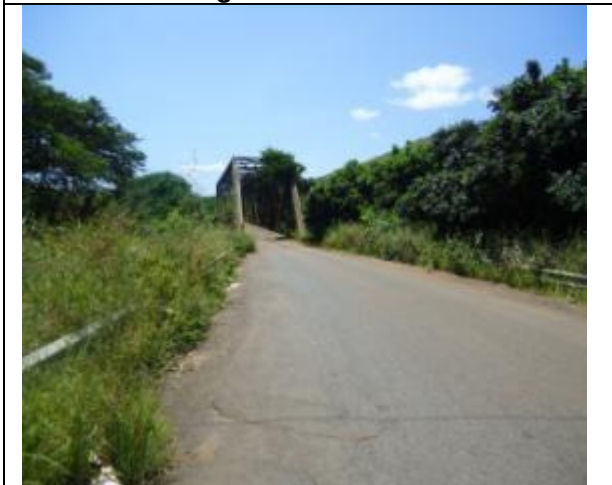
Portion of road before current bridge structure enroute to Nseleni
