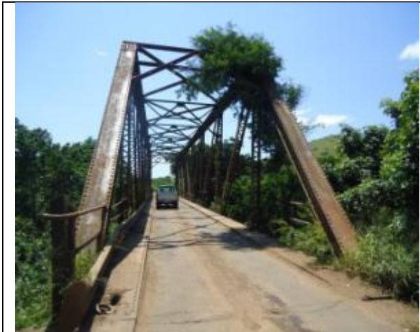
View of the bridge enroute to Nseleni
