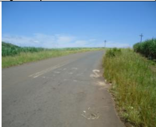
Road from Empangeni to Nseleni before the Current bridge structure
