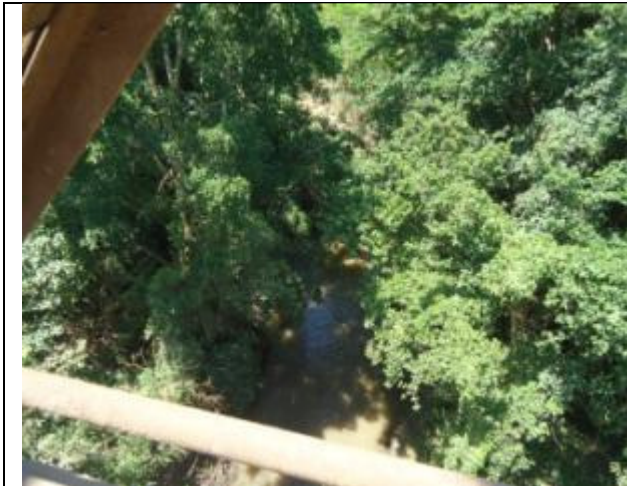
View of Nseleni River downstream from the current bridge structure
