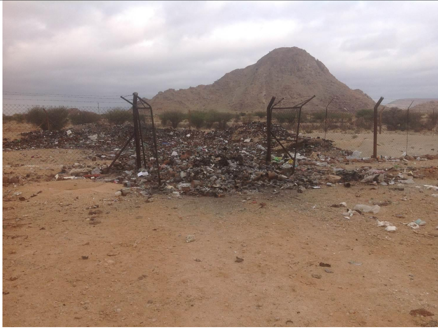
Entrance to the landfill – facing west.
