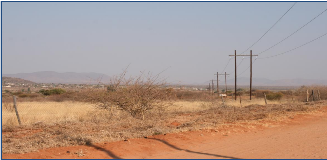
Figure 10: The proposed alternatives will run parallel to the existing power line
