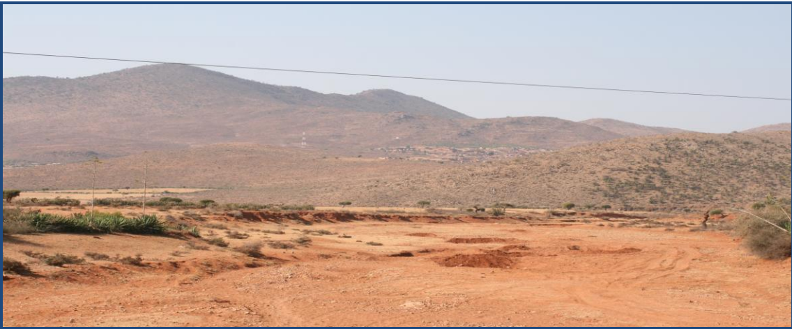
Figure 22: Extent of the erosion at Magobeshane stream
