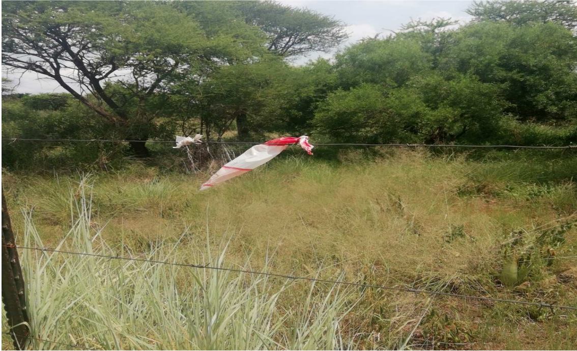
Figure 3: Boundary Fence with a peg showing where the line will be constructed
