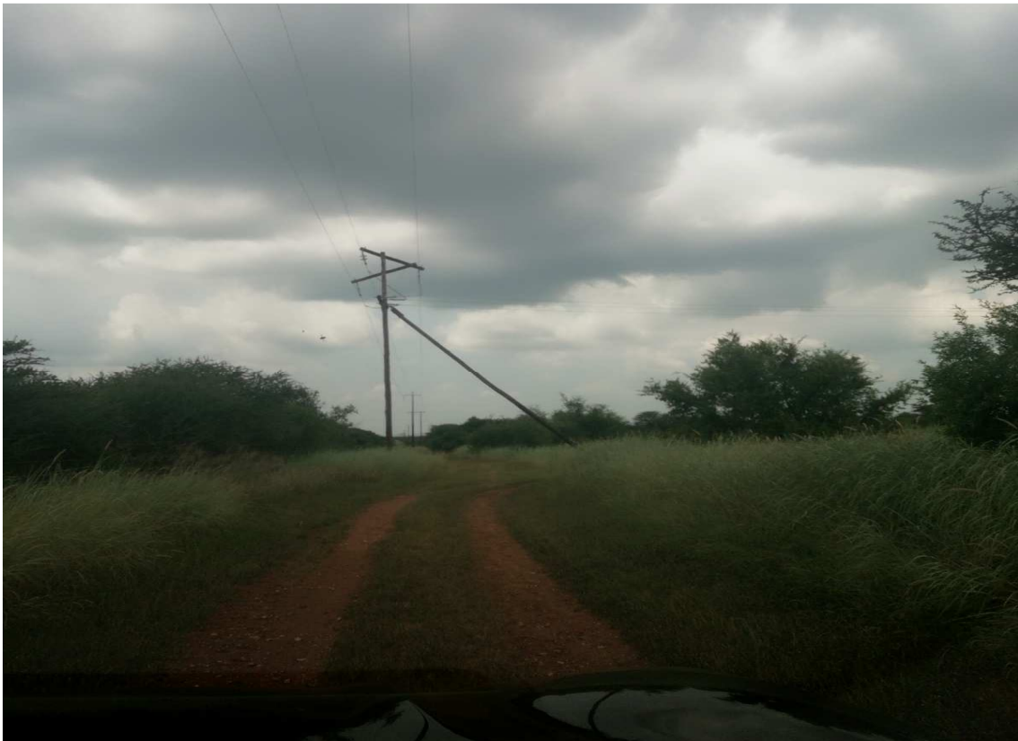
Figure 2: Existing Road and electrical infrastructure
