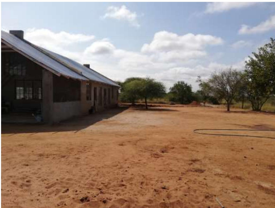
Figure 10 Point of supply
