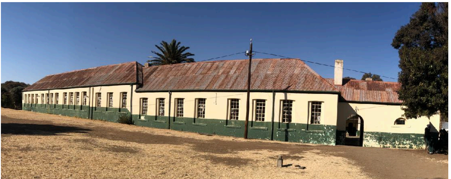
Back Elevations of Existing Buildings - Used as Library & Classrooms
