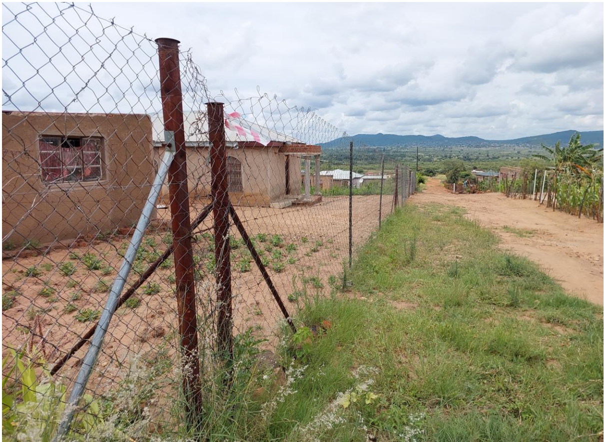
12. Picture no 12 : showing where the power line will be running and peg
