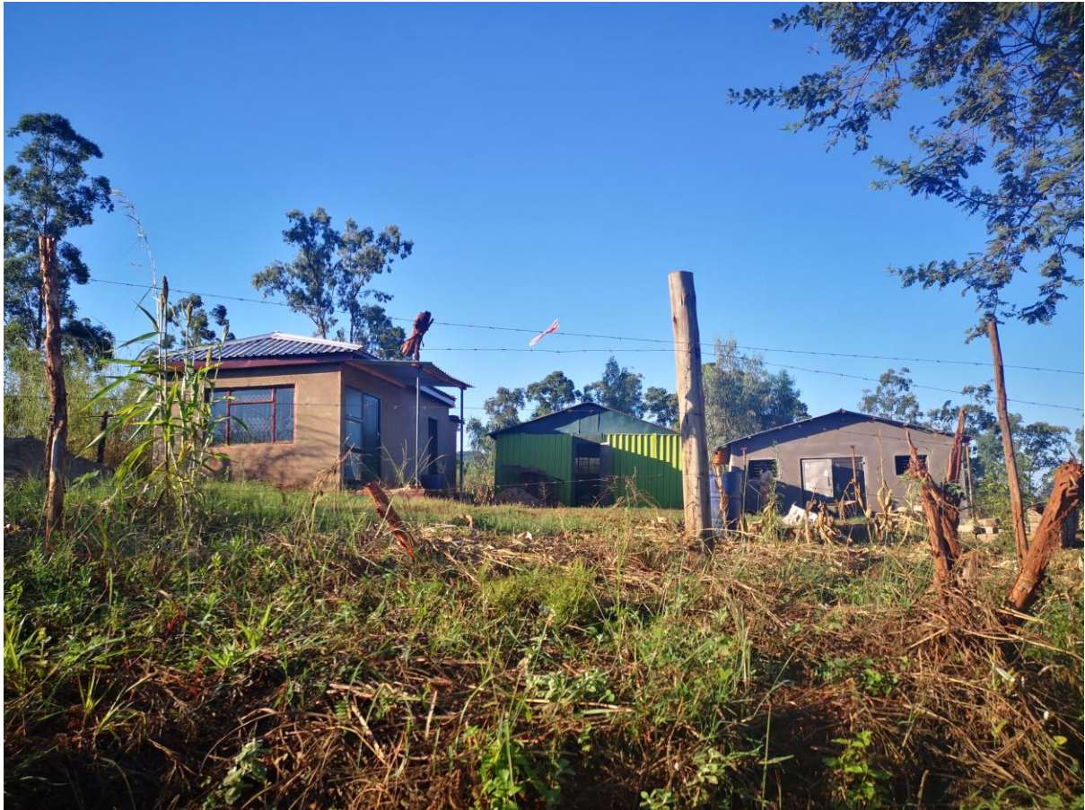
Shows the area where the electricity is required and the peg
