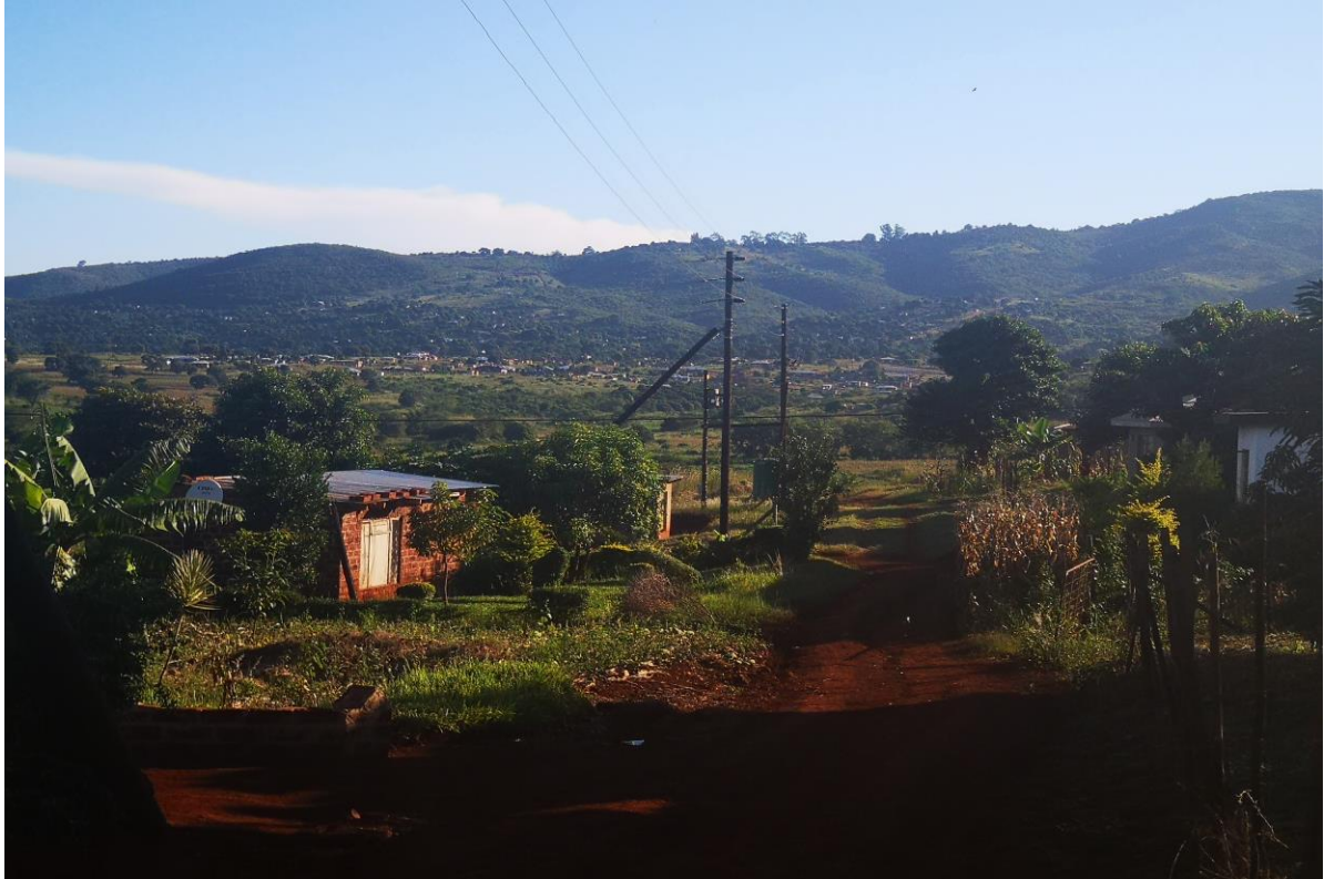
The existing powerline on site
