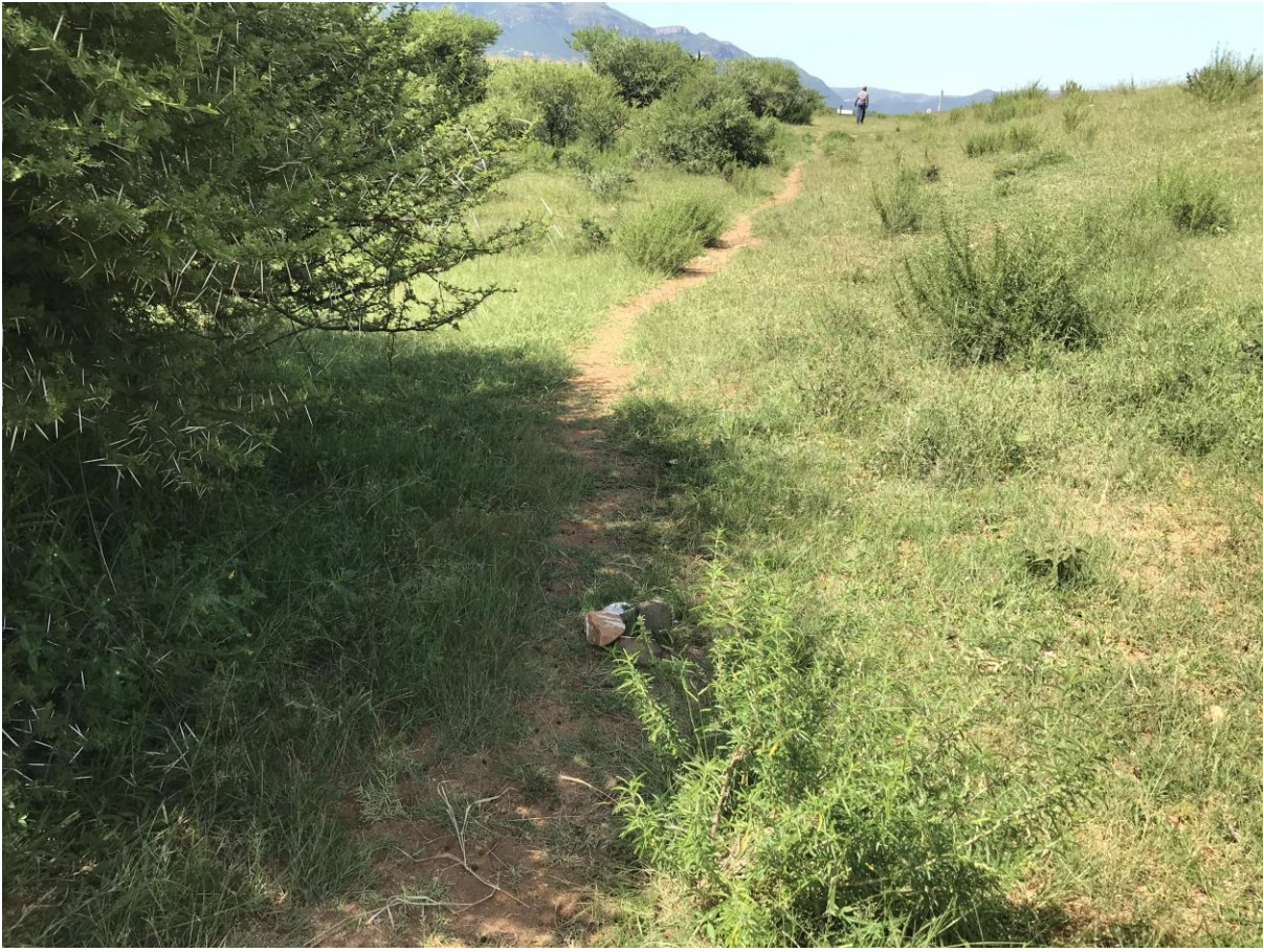
8 Picture no 7: showing the showing where the power line will be running
