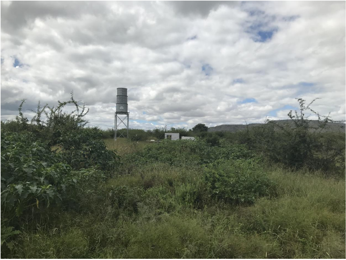
9 Picture no 9: showing the borehole house to be supplied with Electricity
