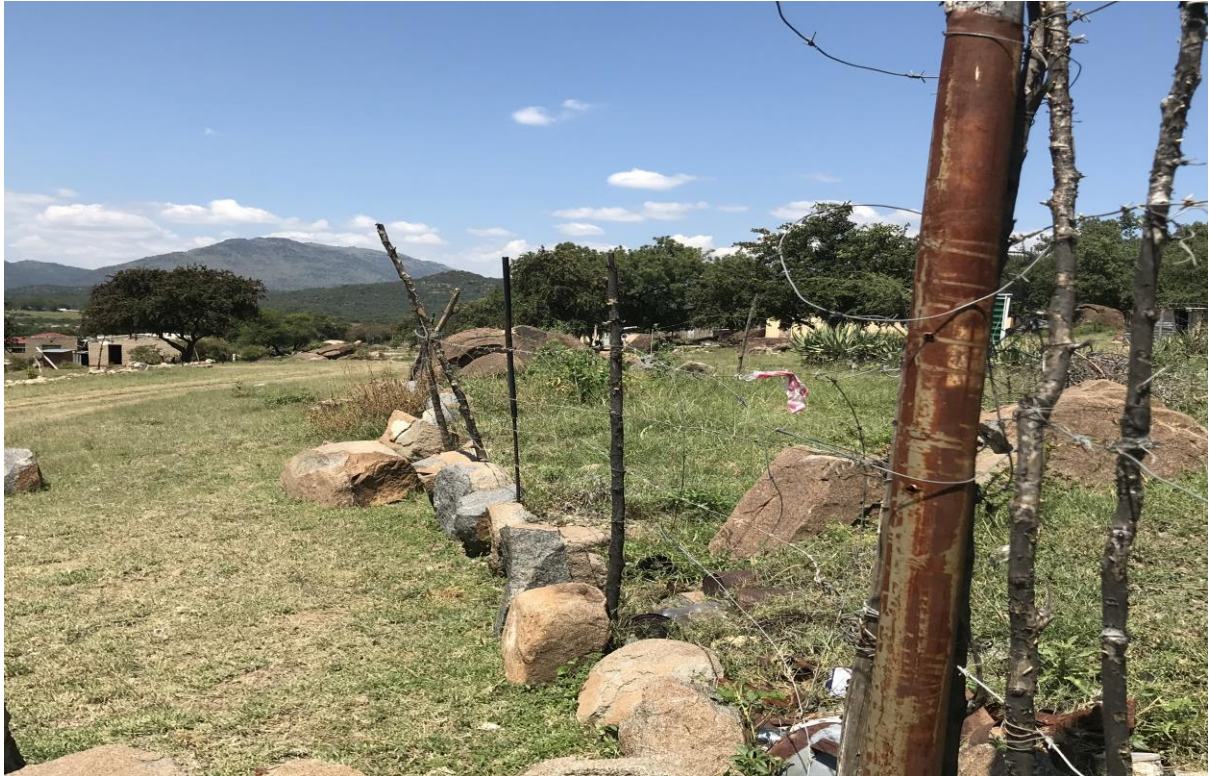
6. Picture no 6 : showing where the power line will be running and peg
