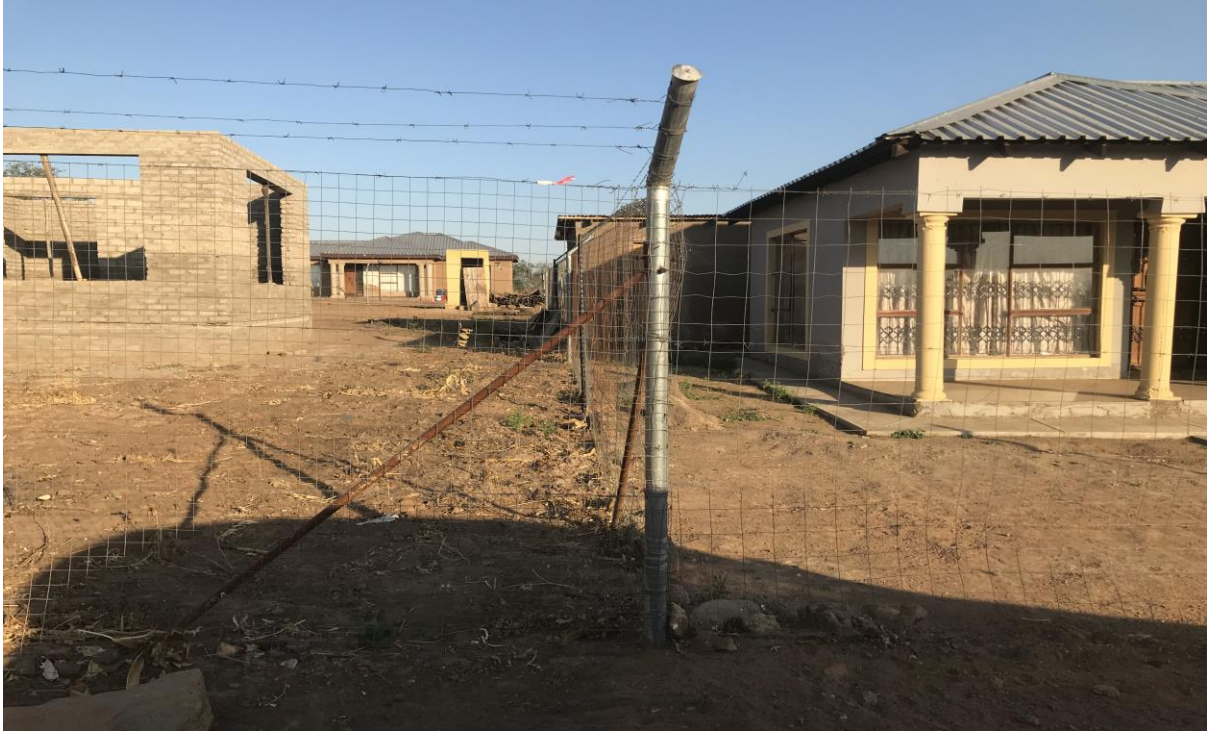
13. Picture no 13 : showing where the power line will be running
