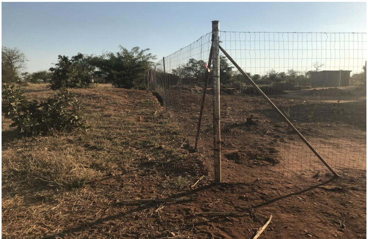
8. Picture no 8 : showing where the power line will be running and peg
