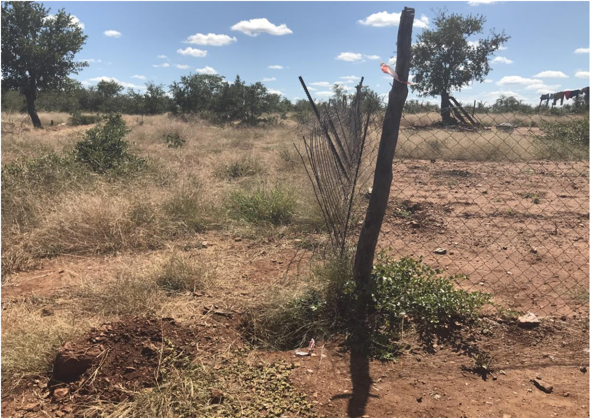
6. Picture no 6 : showing where the power line will be running and peg
