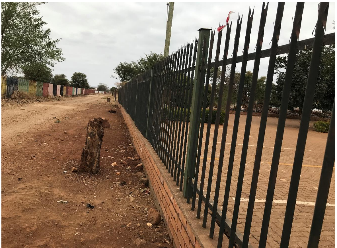
4. Picture no 4: showing where the power line will be running and Existing gravel road.
