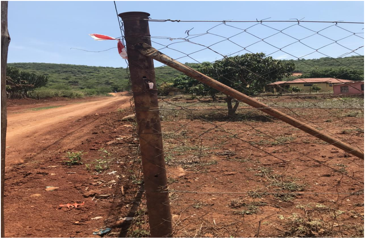
6. Picture no 6 : showing where the power line will be running
