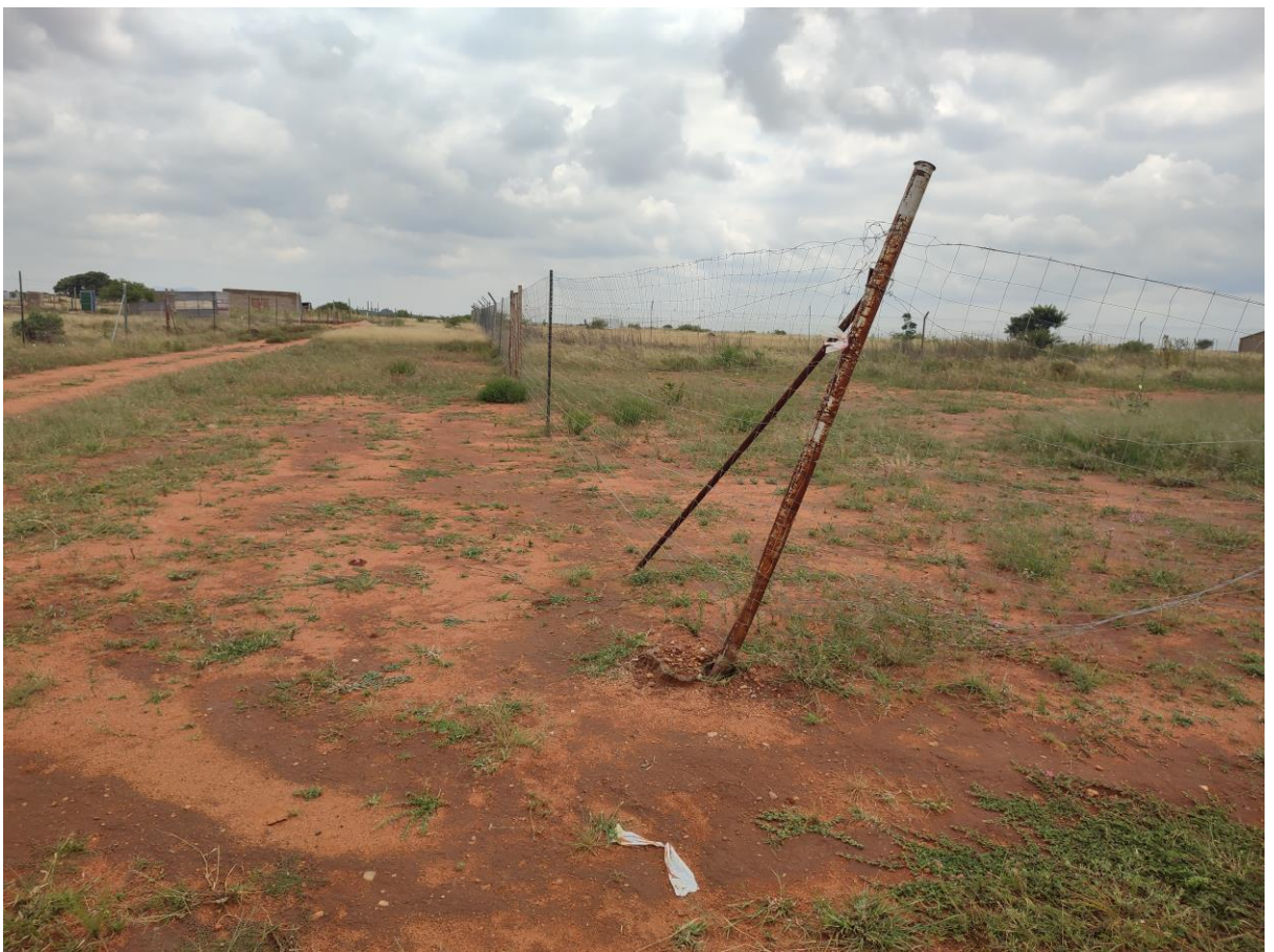
11. Picture no 11 : showing where the power line will be running
