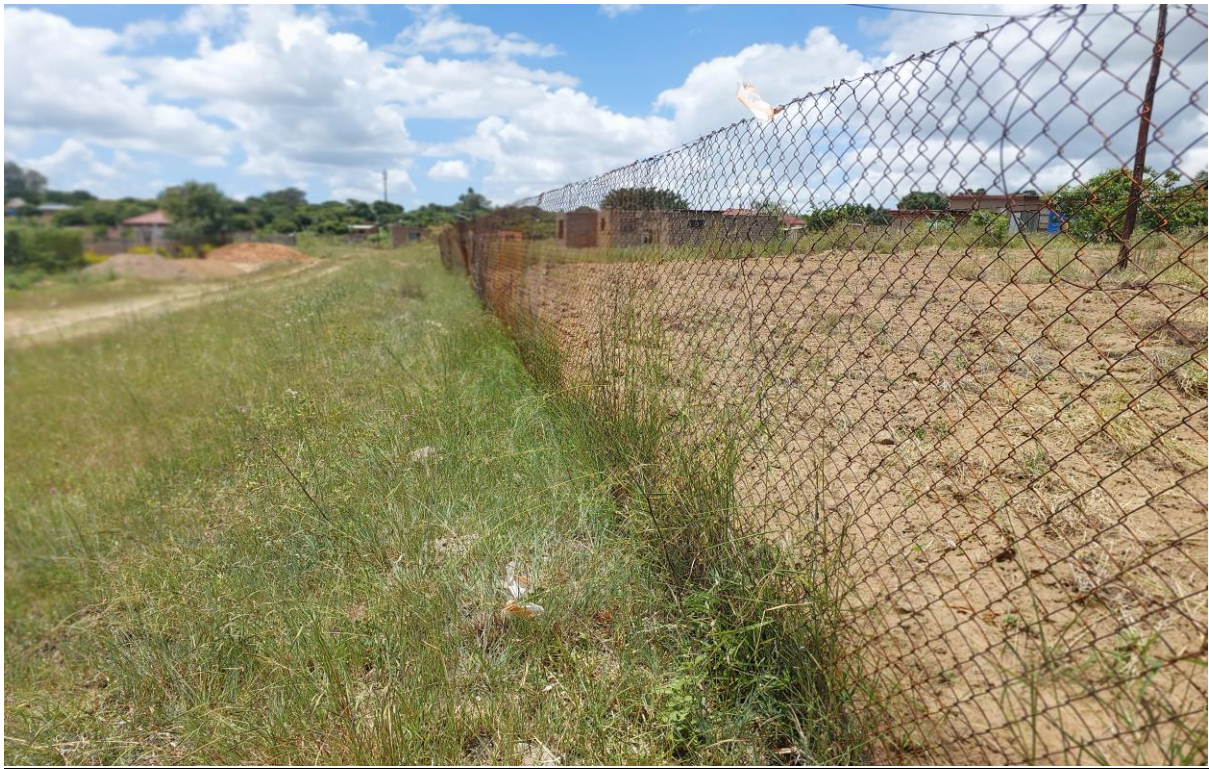
7. Picture no 8 : showing where the power line will be running and peg
