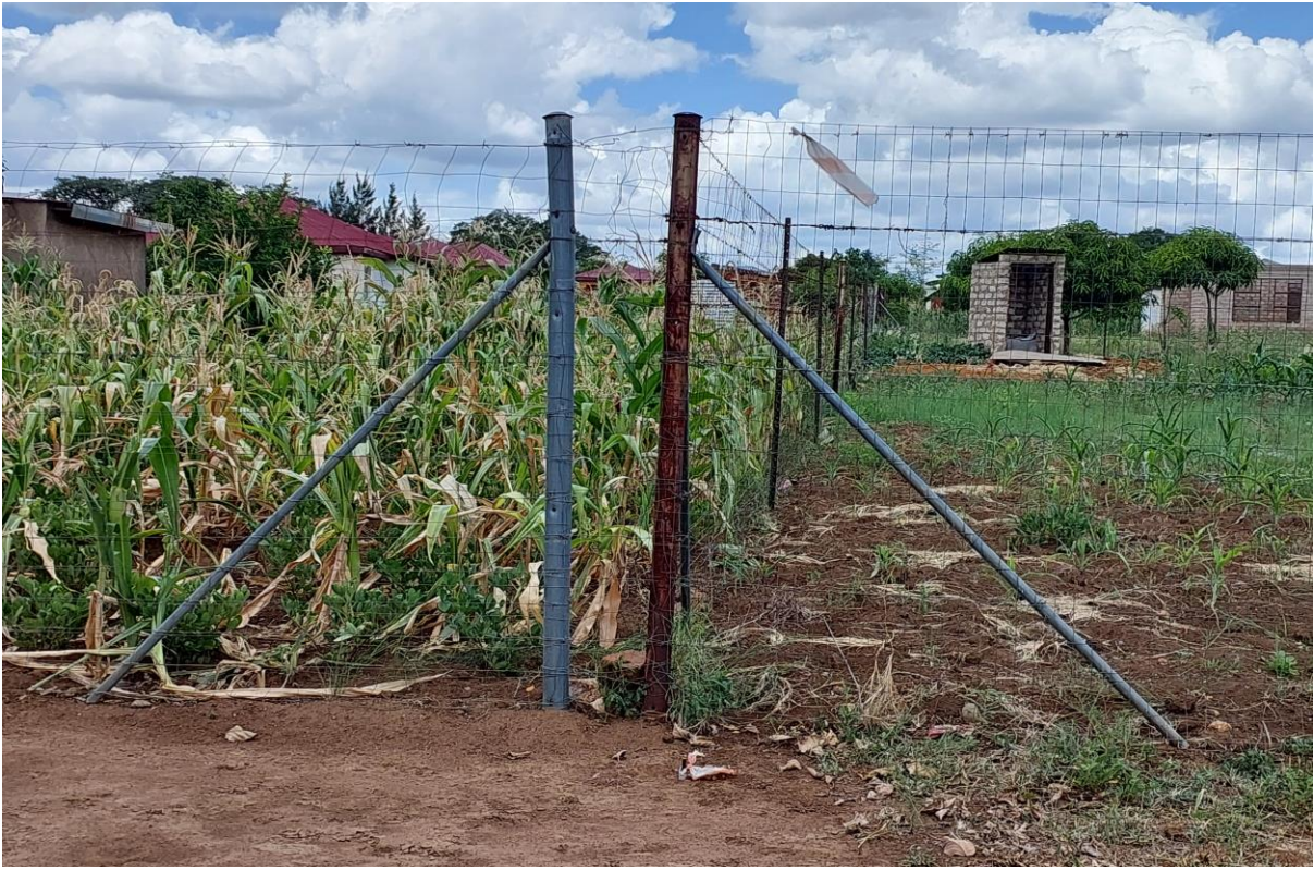
11. Picture no 12 : showing where the power line will be running and peg
