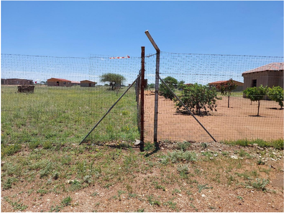
19. Picture no 19 : showing where the power line will be running
