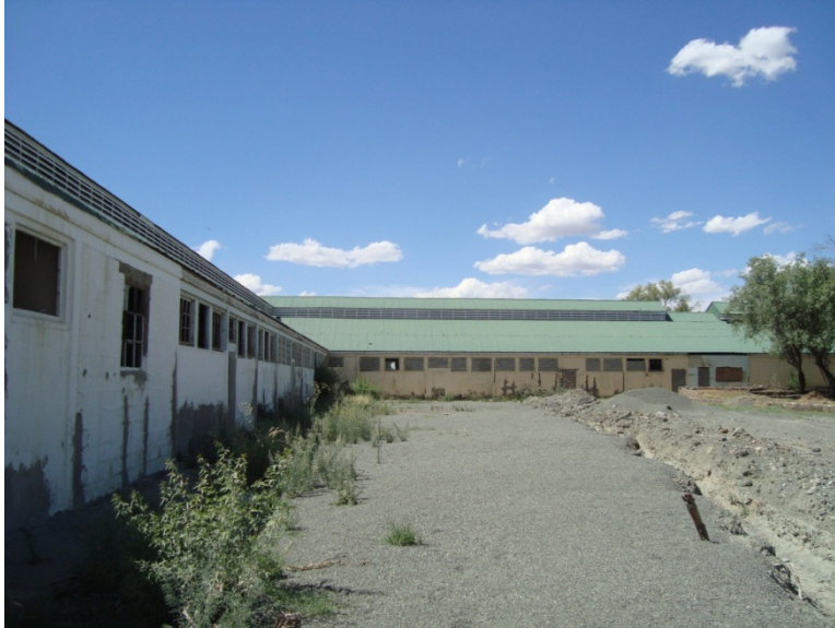
Figure 9. View of the workers' hostel to the north.
