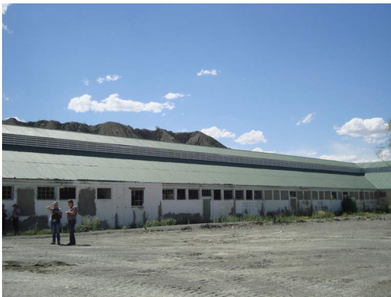
Figure 10. View of the workers' hostel to the northwest.
