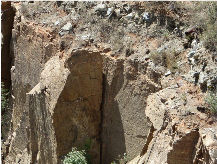
Figure 6. Crack in the side of the mine pit
