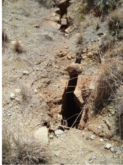
Figure 7. Crack along the perimeter of the mine pit
