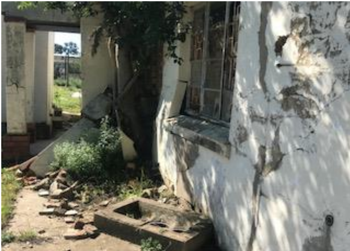
Tree growing in the foundation of Prof Z. K Matthews house in Alice Eastern Cape
