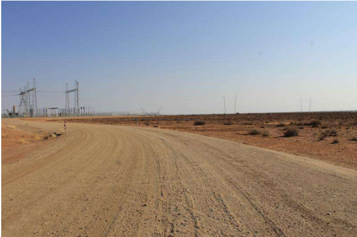
Figure 9 Image of Nieuwehoop substation showing graminoid veld with occasional Acacia - Lyceum associations and individual specimens.
