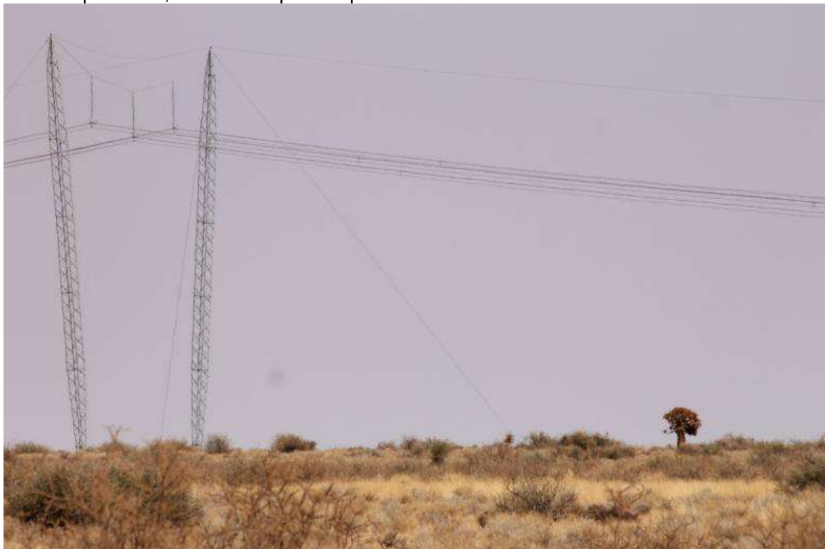
Figure 7 Image showing existing powerline near Skeerhok Alternative 1, with A dichotoma present in close proximity to tower.
