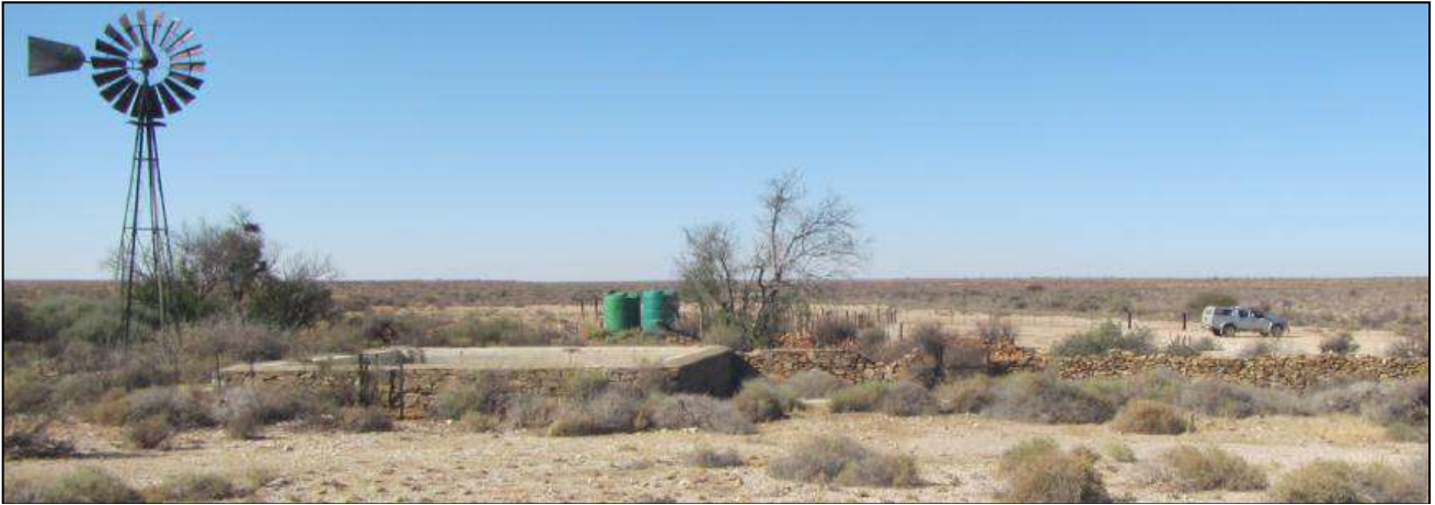
Figure 37: Stone reservoir with a recent cement lining, wind pump, drystone walling and two modern water tanks. The wind pump had been decommissioned (waypoint 849).
