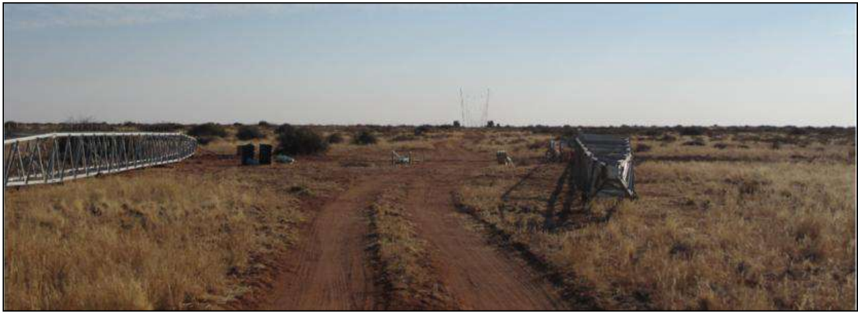
Figure 7: View northwards along the north-western margin of the study area showing a new power line currently under construction (during July 2017) parallel to part of Alternative 1.
