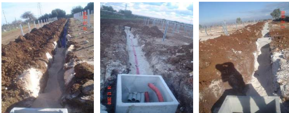
Figure 8: Cable trenches
