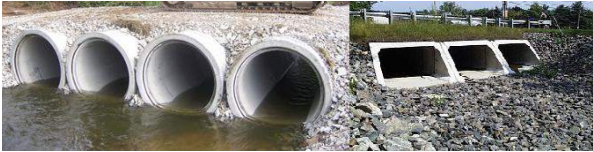
Figure 18: Installed concrete pipes and culverts
