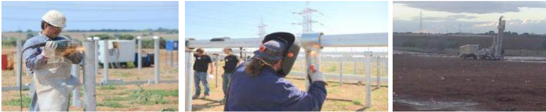
Figure 12: Onsite construction of the PV arrays
