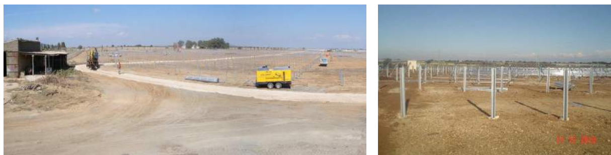
Figure 11: Illustration of a typical site after preparation
