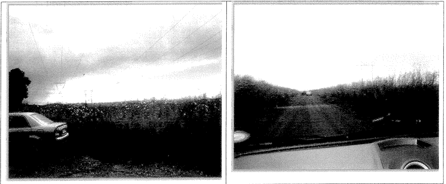
Plate 2: Existing access road and the powerlines
