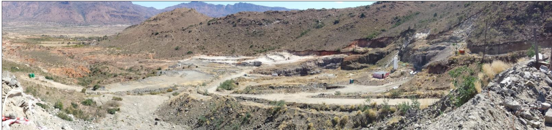
Figure 3: View of the opencast and underground mining area between Hills 2 and Hill 3 looking south-west.
