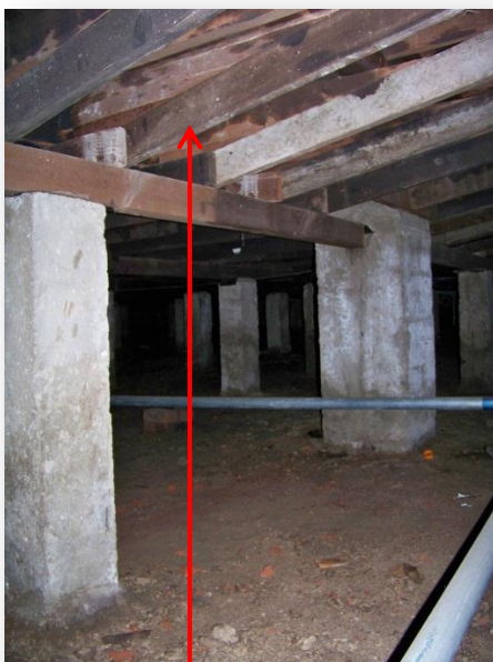
Floor boards on top of support pillars.
