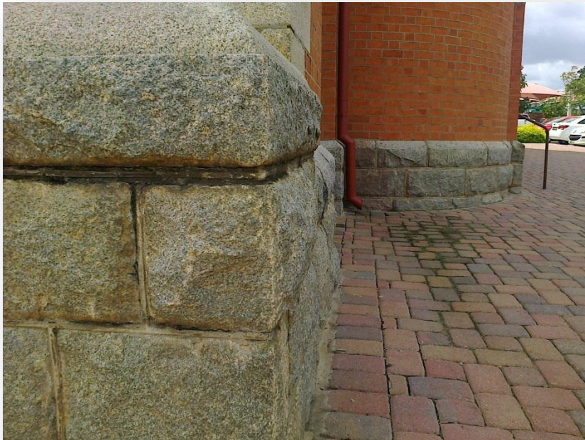
Exterior of the granite foundations.
