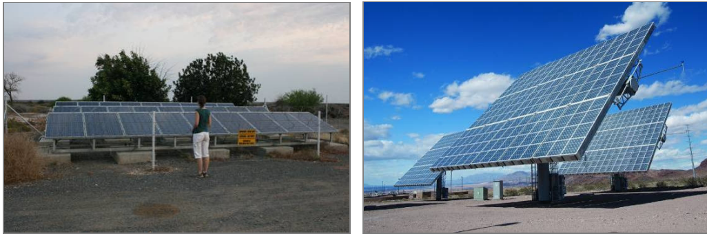
Figure 2.7: Photovoltaic solar cells (left) 24 and a CPV system (right) 25 were considered for the proposed PV plant
