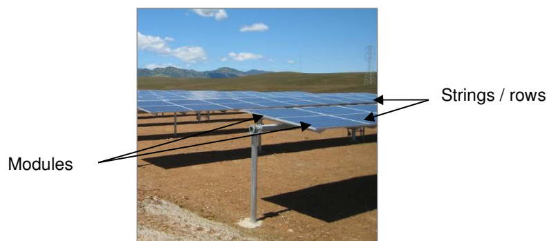
Figure 2.2: Typical layout of panel structures
