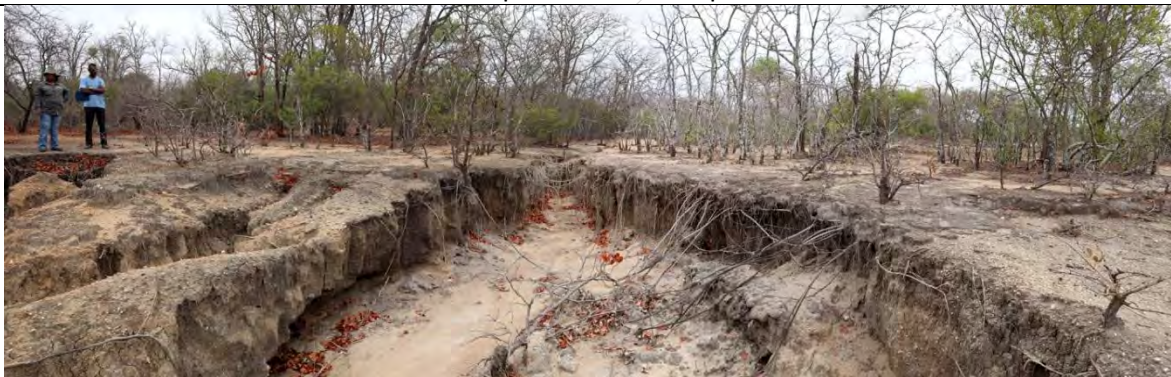
Head-cut erosion in the downstream portion of the wetland
