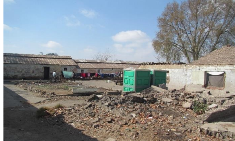
View showing some of the brick buildings in the compound
