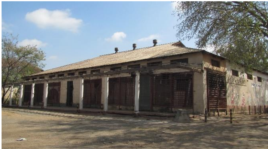
View of the front of the old shop building
