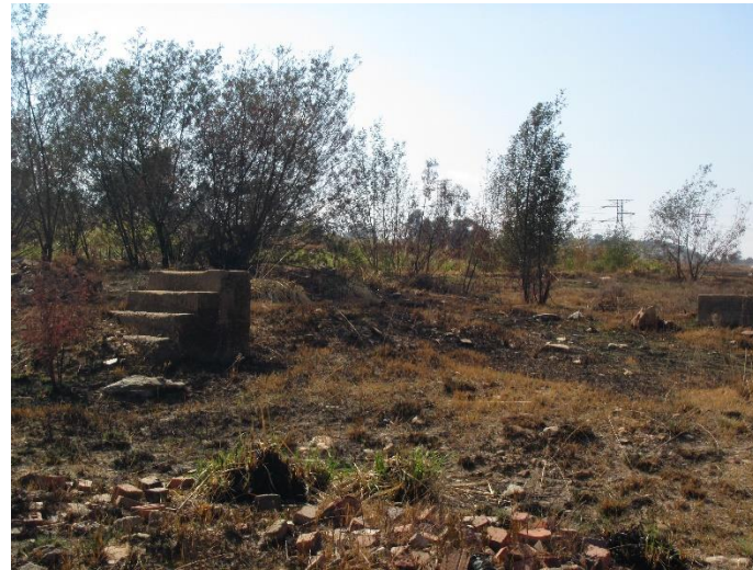
View of the stairs and scattered rubble
