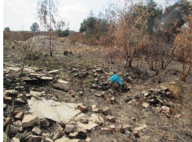
View of building rubble
