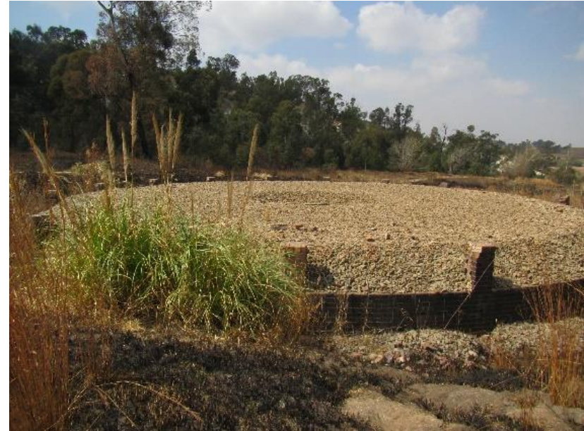
View of the circular base for a reservoir
