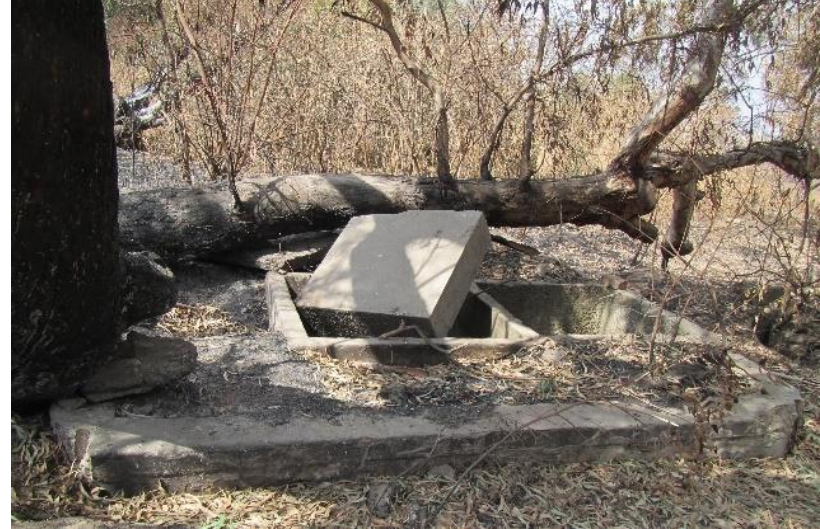
View of one of the structure remains
