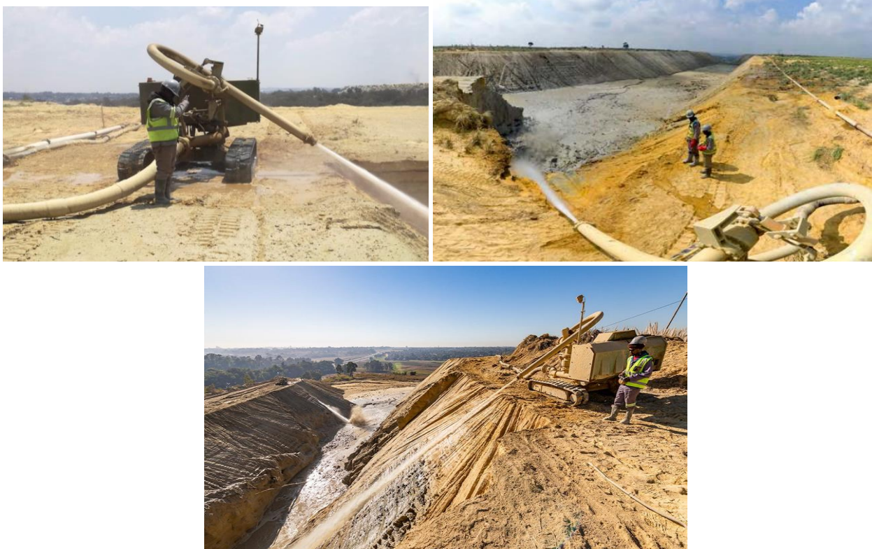
Figure 2-2: Mobile tracked hydraulic monitor on a tailing's facility in South Africa
