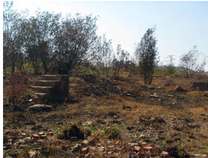
View of the stairs and scattered rubble
