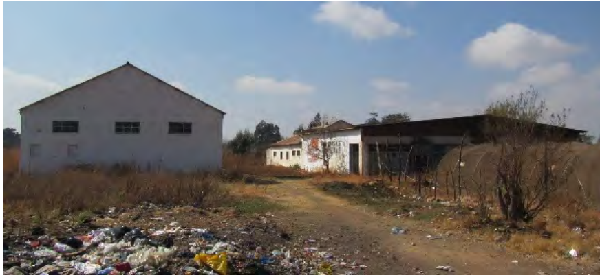
View of the buildings outside the old compound
