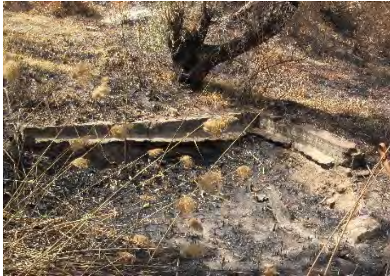
View of one of the structure foundation remains
