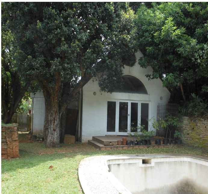
Existing pool house and pool on lower level.
