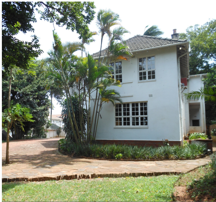
Side of existing house and driveway on upper level.
