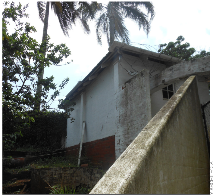
Existing Caretakers House
