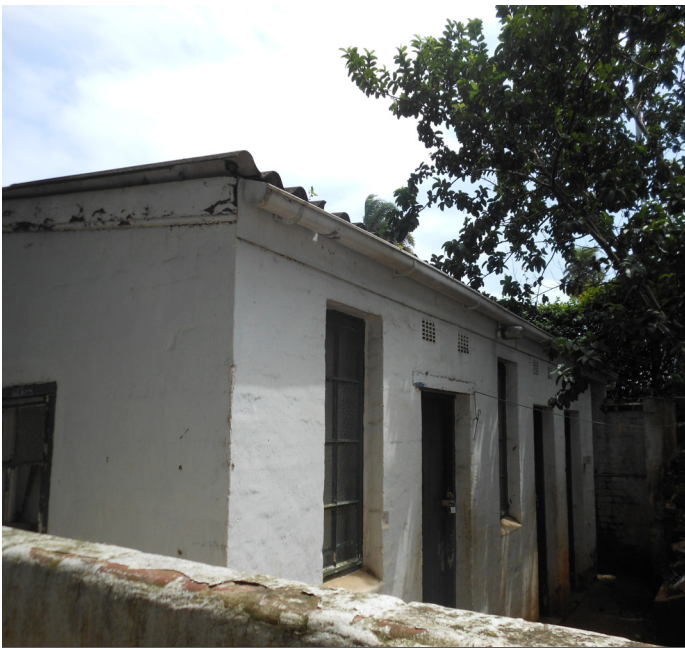
Existing Caretakers House
