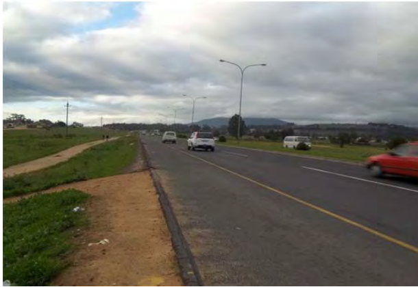
Photo 1: Northbound view on the Western side of Jan van Riebeeck Drive
