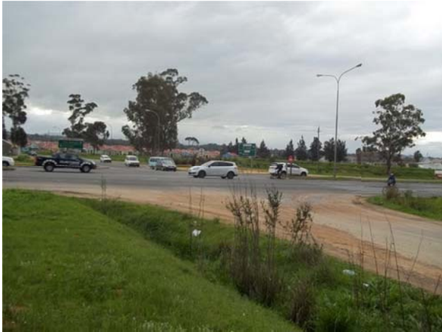
Photo 1: Roggeland Road / Jan van Riebeeck Drive intersection.
