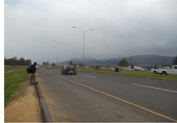
Photo 2: Southbound view on the Eastern Side of Jan van Riebeeck Drive
