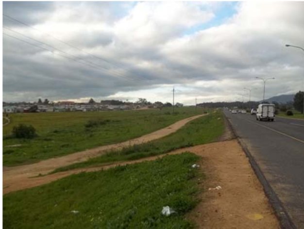
Photo 3: Informal Pedestrian pathways west of Jan van Riebeeck Drive
