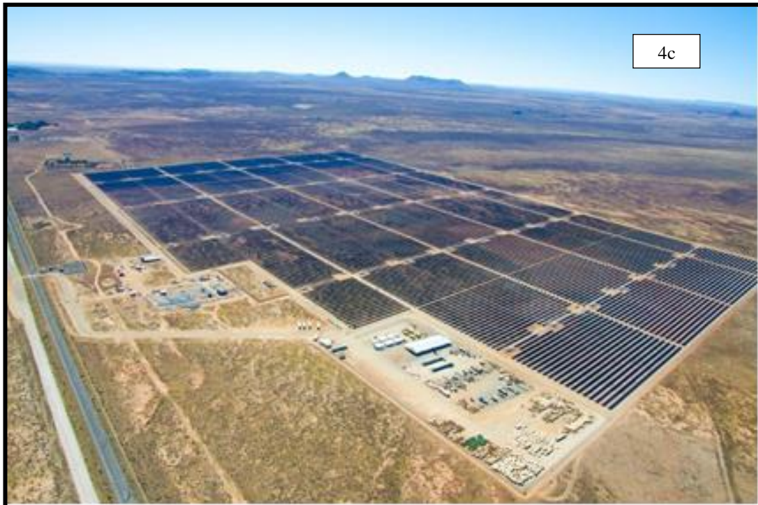
Fig. 4 c Aerial image of Kalkbult solar park, Northern Cape
