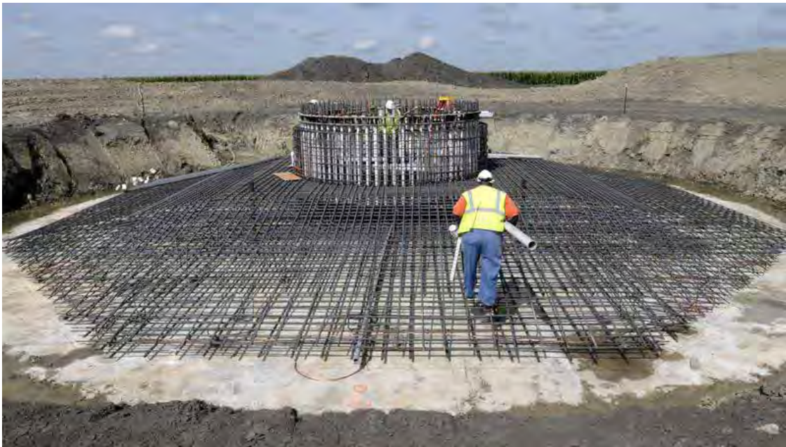
Figure 7.3: Photograph illustrating the construction of the foundation for a wind turbine 9
