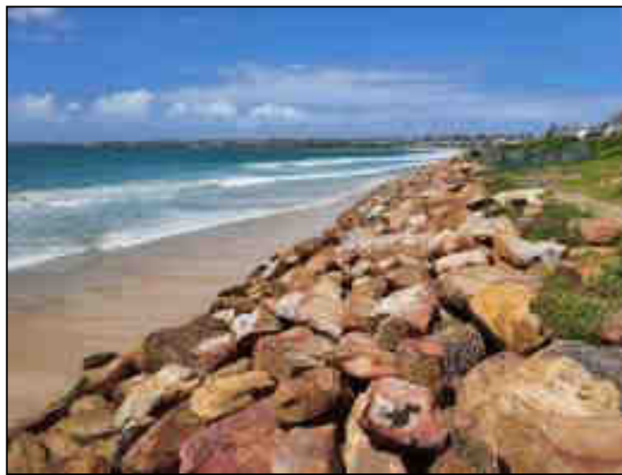
Figure 3-1: View of extensive rock revetments along the coast line.
