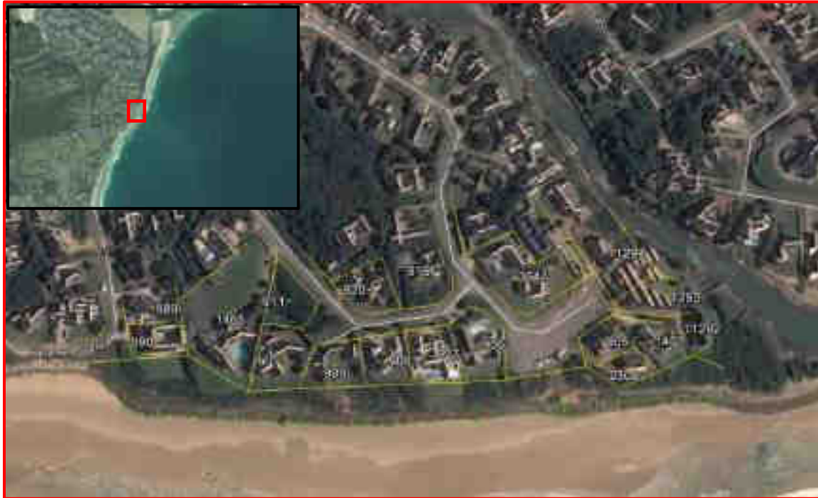
Figure 3: Location of revetment upgrade (PRDW, 2015)
