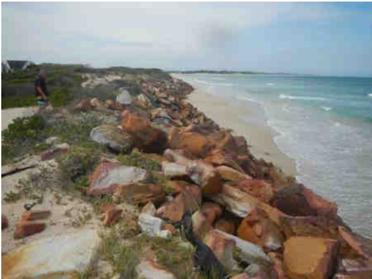
Plate 6.3 Shoreline in the vicinity of Ralph Road, with rock revetments along the HWM (2019). Note the entire absence of a foredune, and wave run-up to the toe of the revetments, due to complete erosion of the foredune and back-beach.
