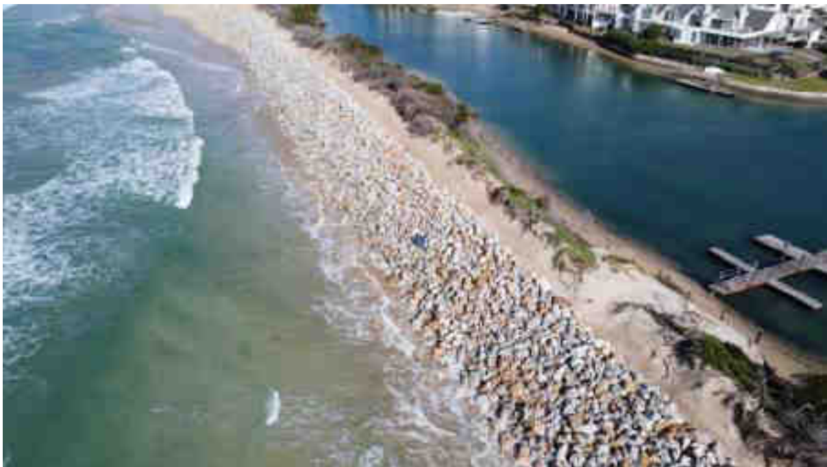
Plate 6.9 Completed revetment along 600 m of the Spit (SFPO NPC)
