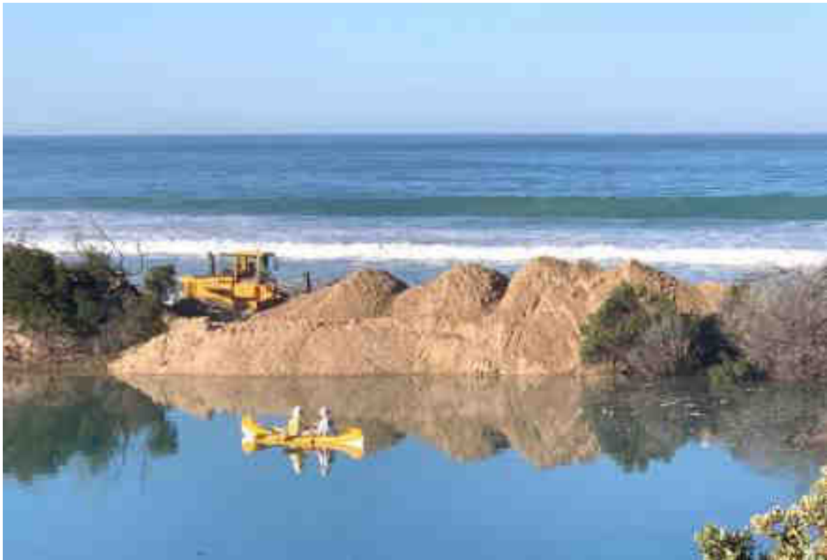
Plate 6.6 A repair of the spit in progress with beach material used for the repair (SFPO NPC)
