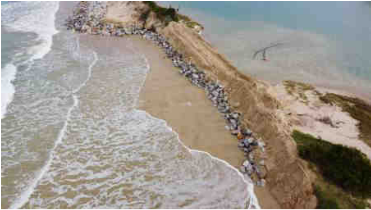
Plate 6.8 Spit repair with sand material and initial rock protection (SFPO NPC)
