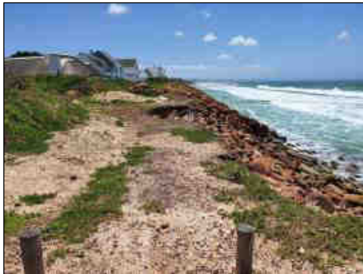
Figure 3-7: View of residential houses and vegetated coastal dunes along rock revetments.
