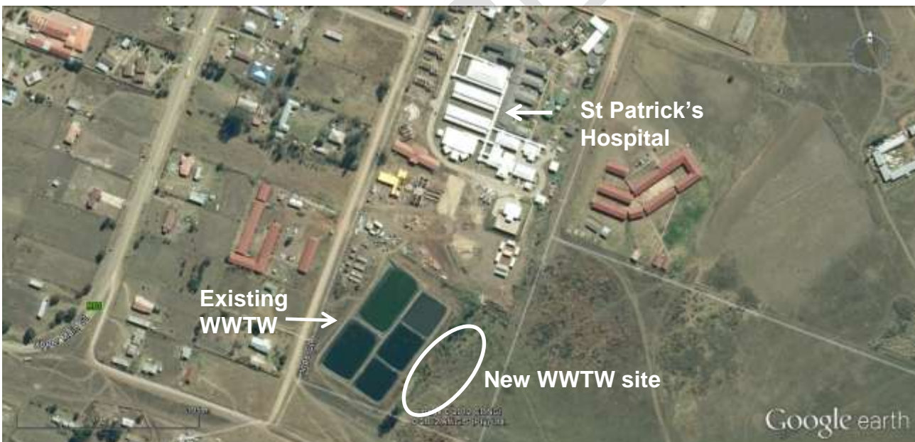
Figure 2.2 Locality of the existing and proposed new WWTW facility for St Patrick's Hospital. The current oxidation pond system is indicated by the orange outline.
