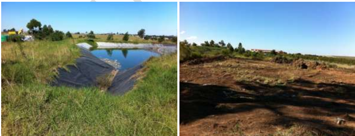
Figure 4.4 Onsite vegetation (top) and excavated site (bottom).
