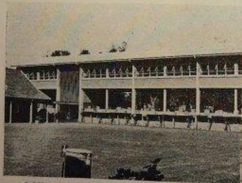
Addition of 5 classrooms to the new block commence.
