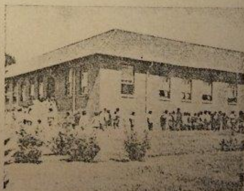
Part of the original building.
