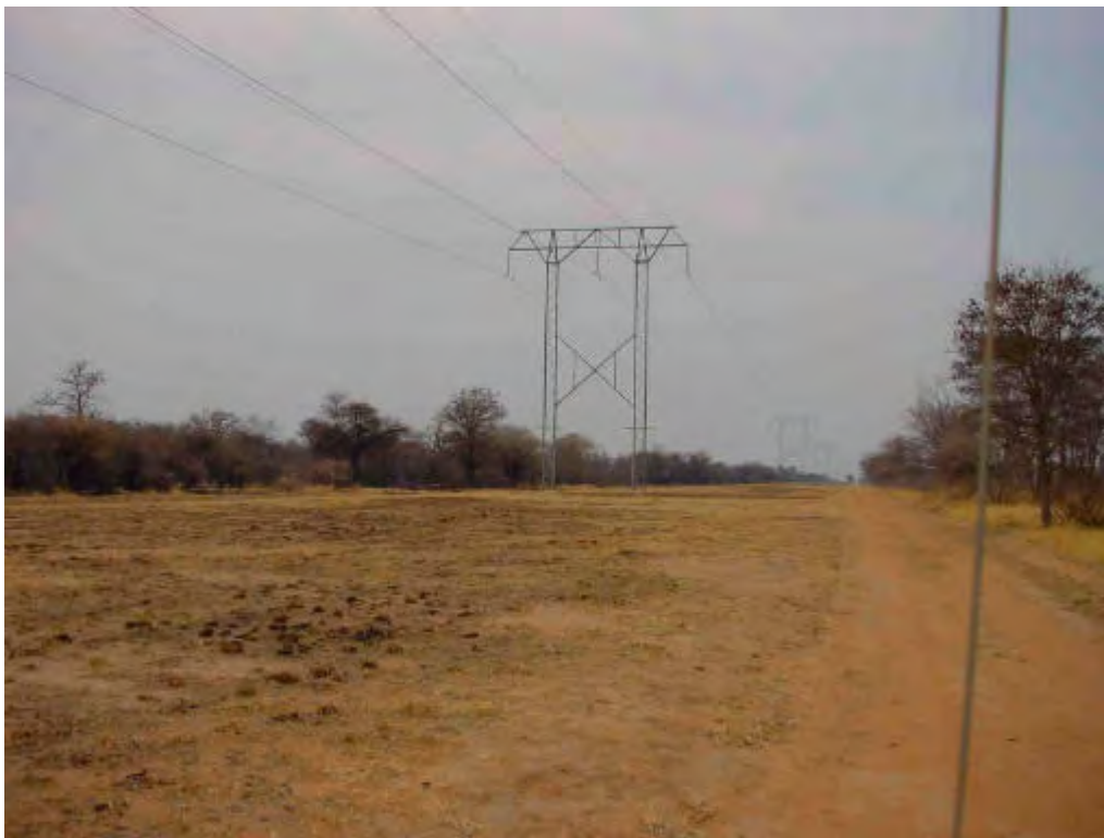
Figure 7. Example of a power line servitude used as a fire break at Thaba Tholo near Thabazimbi.
