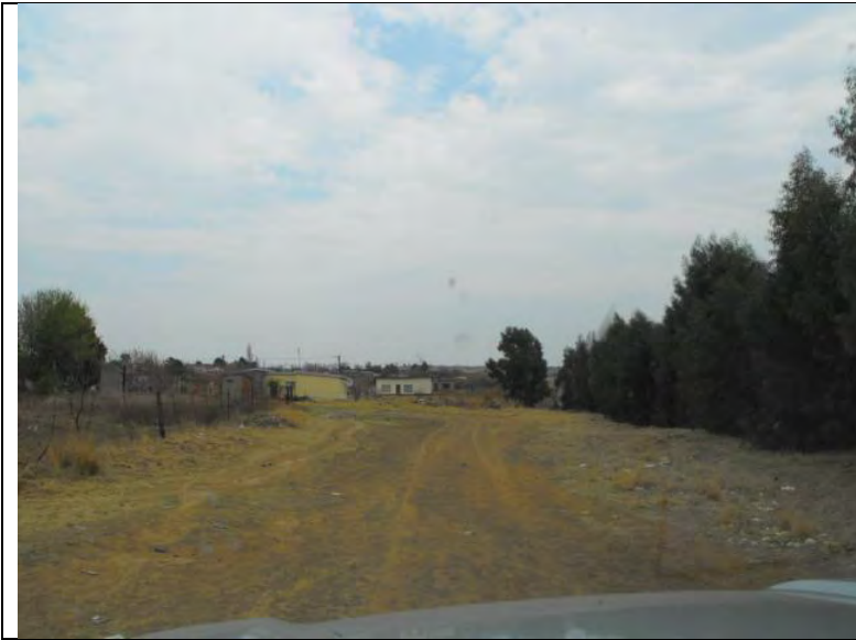
Figure 13: View of the Phase 2 pipeline along the western split. The pipeline will be installed adjacent to the road.
