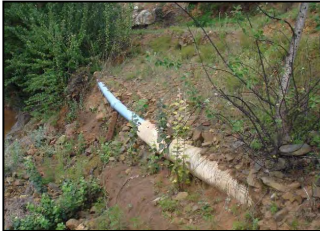
Figure 14: AC sewer pipe repair with smaller PVC
