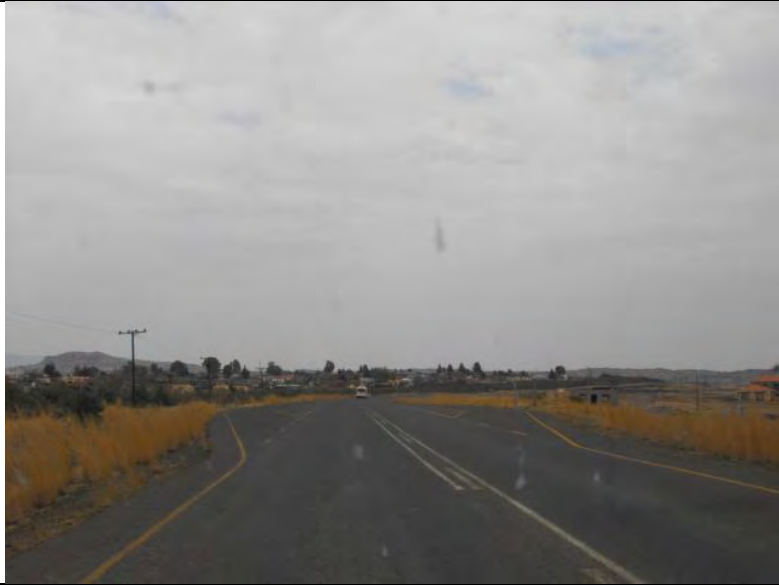
Figure 12: View of the Phase 2 pipeline along the western split. The pipeline will be installed adjacent to the road.
