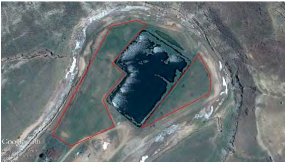
Figure 1: Existing maturation ponds with the surrounding areas where the final effluent was previously irrigated.
