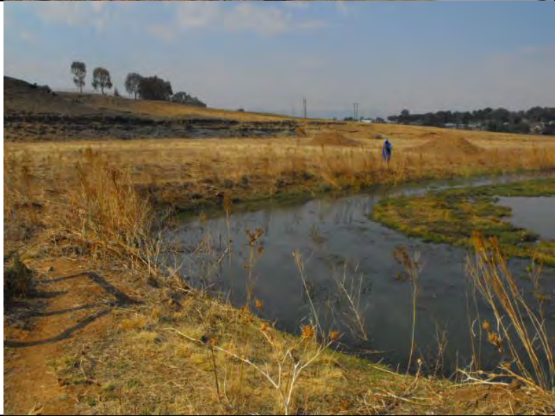
Figure 3: View of the WWTW toward the south. The existing oxidation ponds are visible.
