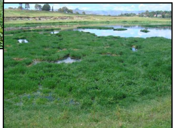
Figure 12: Overgrow in oxidation pond
