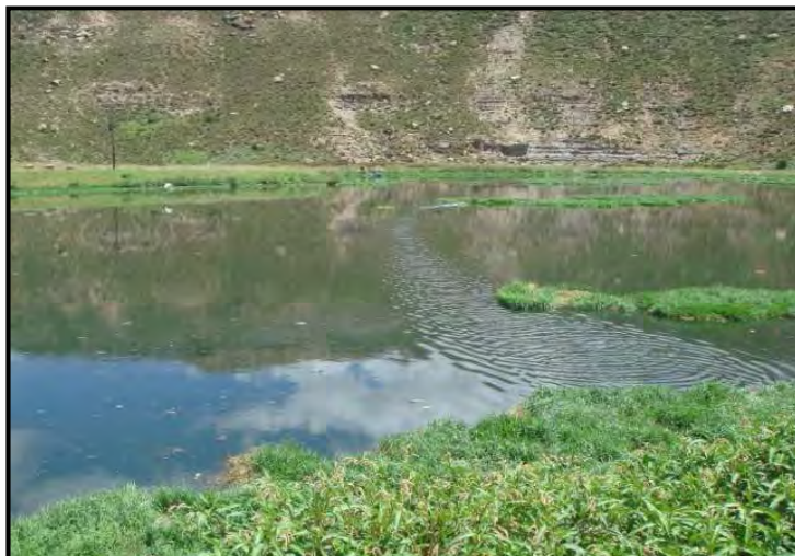
Figure 13: Oxidation pond full to capacity
