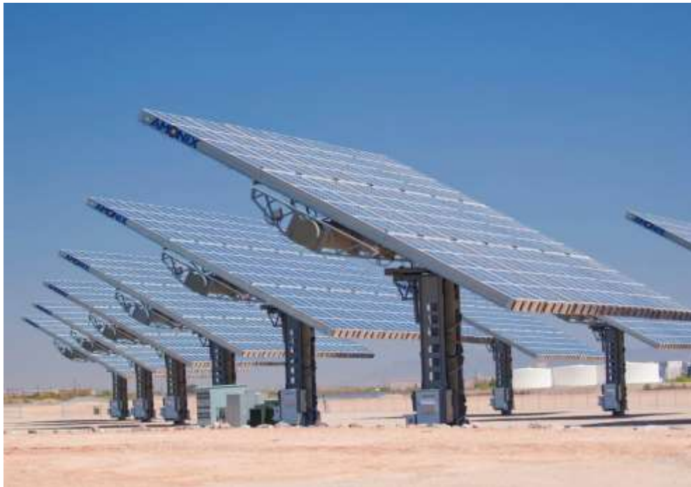
Figure 2.10: The support structures elevate the panels by 15 m and allow for dual axis tracking of the sun for increased efficiency (Source of Amonix™)
