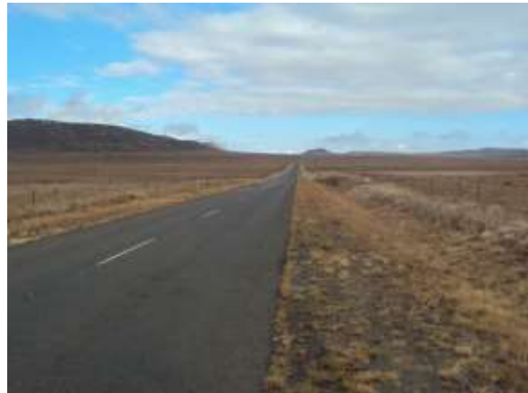
Figure 2.4: View of the R56 in the direction of Molteno
