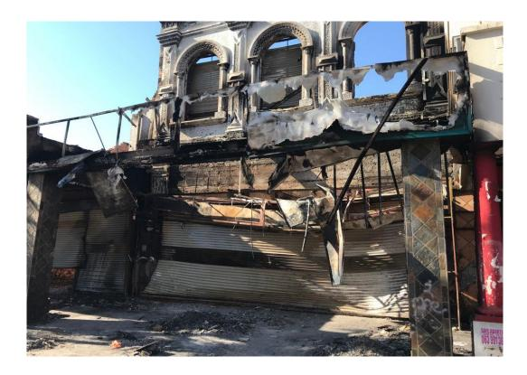
2. The brick rubbles and the roof resulted in structural collapse to damage the internal floor.
