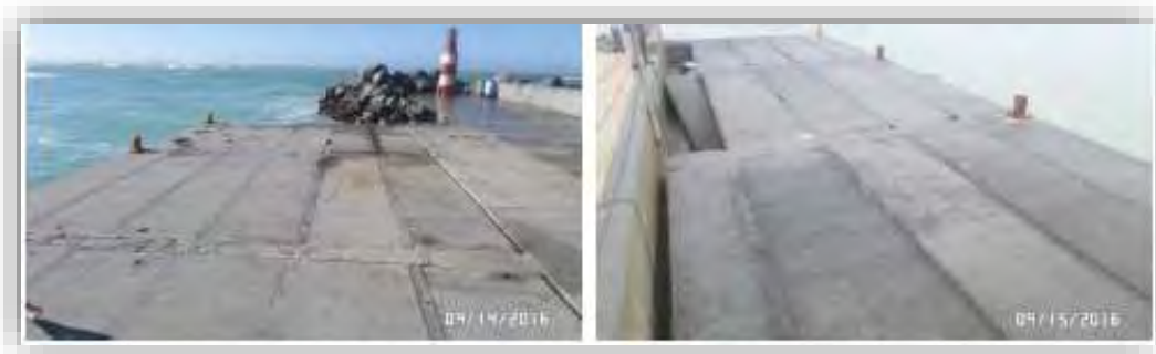
Figure 3: Quay 1 (left) and Quay 2 (right)
