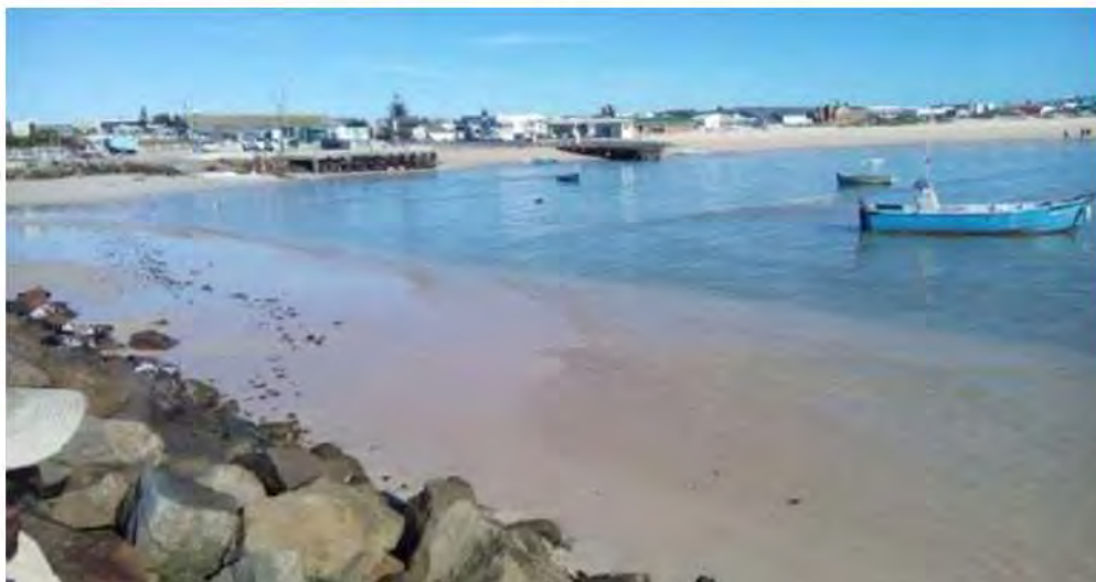
Figure 2: Struisbaai harbour – sediment build-up
