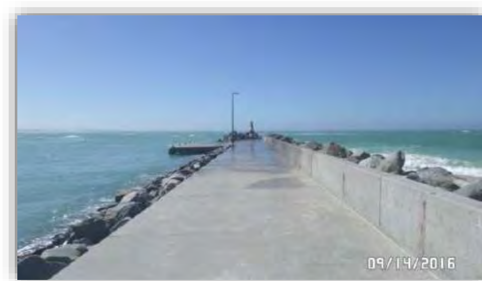
Figure 2: Struisbaai harbour breakwater.
