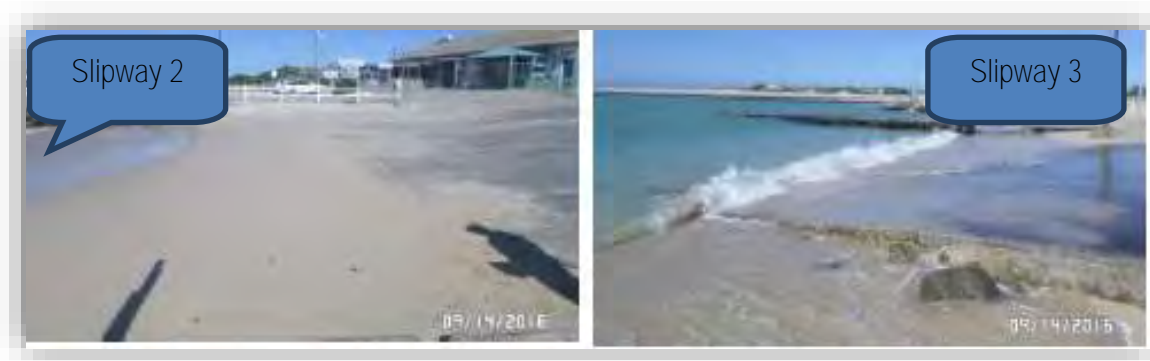
Figure 5: Slipways 2 and Figure 6: Slipway 3
