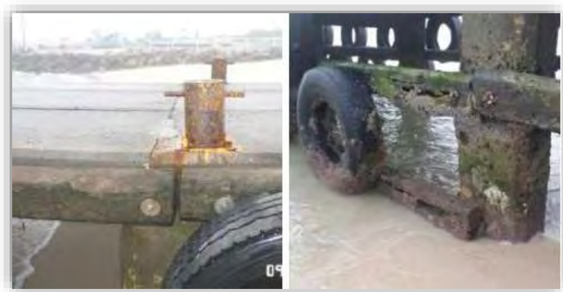
Figure 8: Bollards and timber
