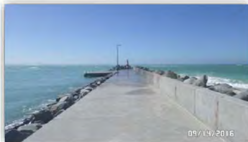
Figure 5: Struisbaai harbour breakwater
