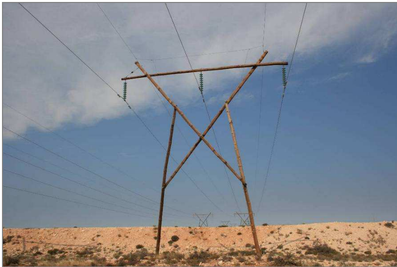
Figure 2.2 Example of an existing 132 kV transmission line onsite (taken 29/09/2011)
