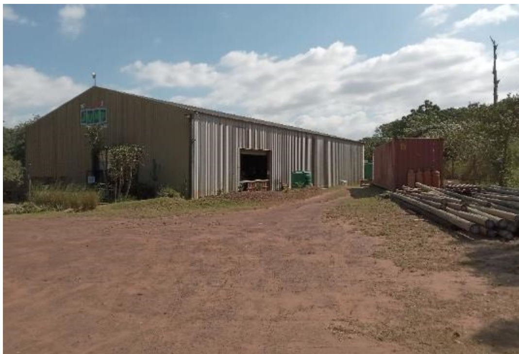
Figure 20: Structure and parking lot on northern boundary of the site
