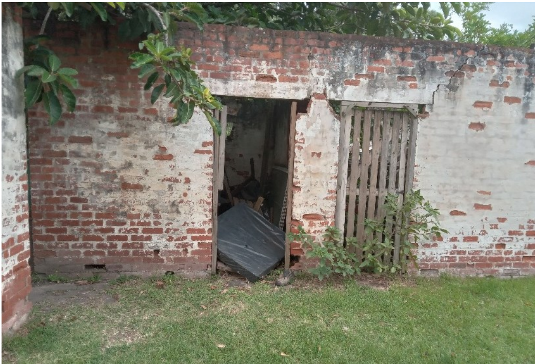
Figure 12: Structure in compound
