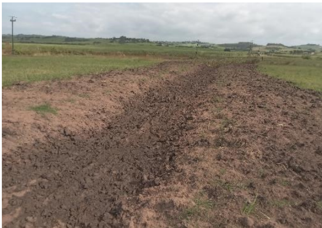
Figure 19: Cleared drainage line
