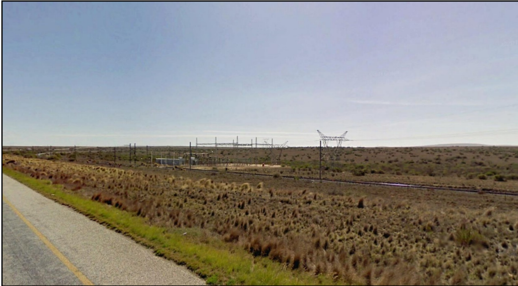
Figure 7: The Rippon Substation as seen from the N10 national road.
