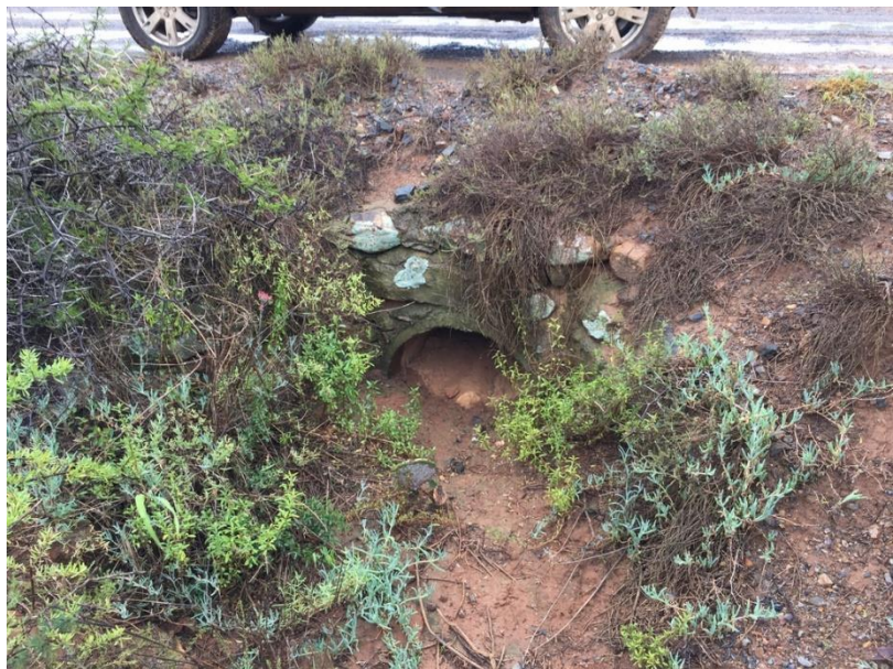
Figure 4 – Stormwater Crossing along DR02054
