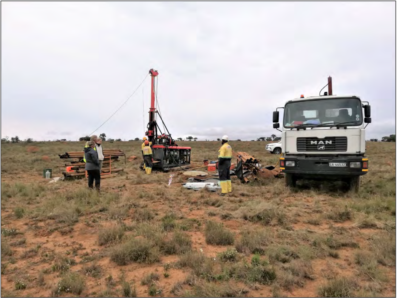
Plate 1: Rotary core drilling at borehole position E64
